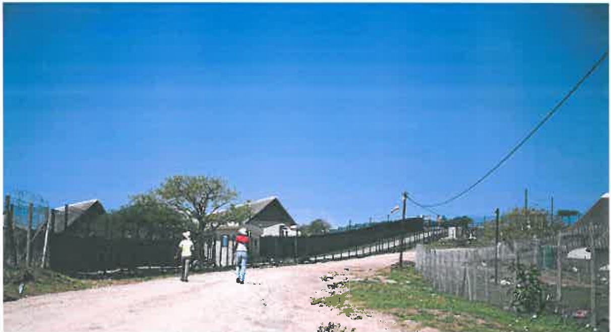
Lie of the land: Phase one, which included road and fence upgrades, bypassed departmental guidelines to favour Zuma's personal choice of contractors. Photos: Madelene Cronjé
