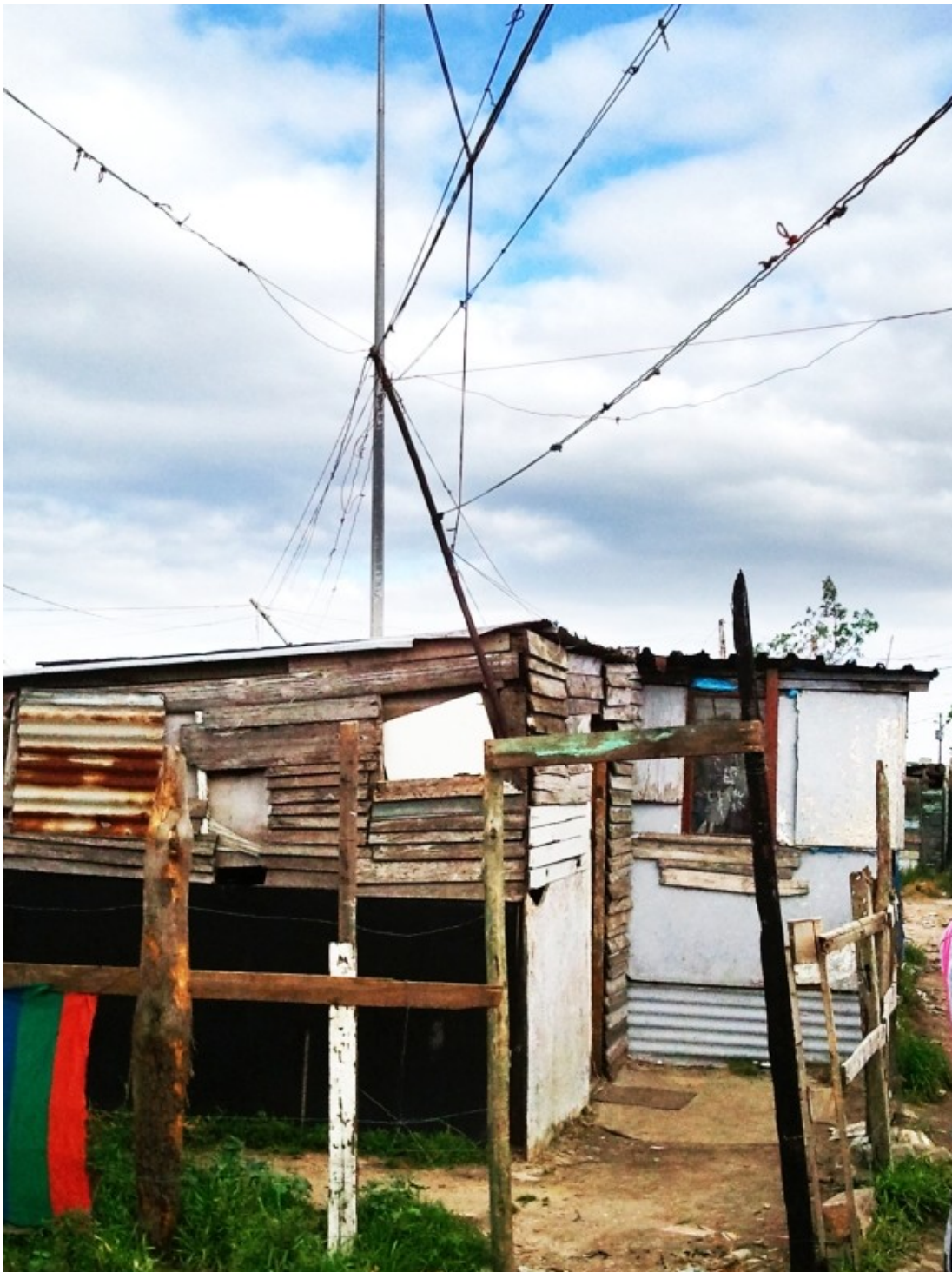
Sweet Home's anti-shackfire strategy: informal electricity connections
