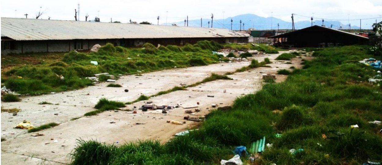
Adjacent private property that is blocking and further polluting Sweet Home's sewage system
